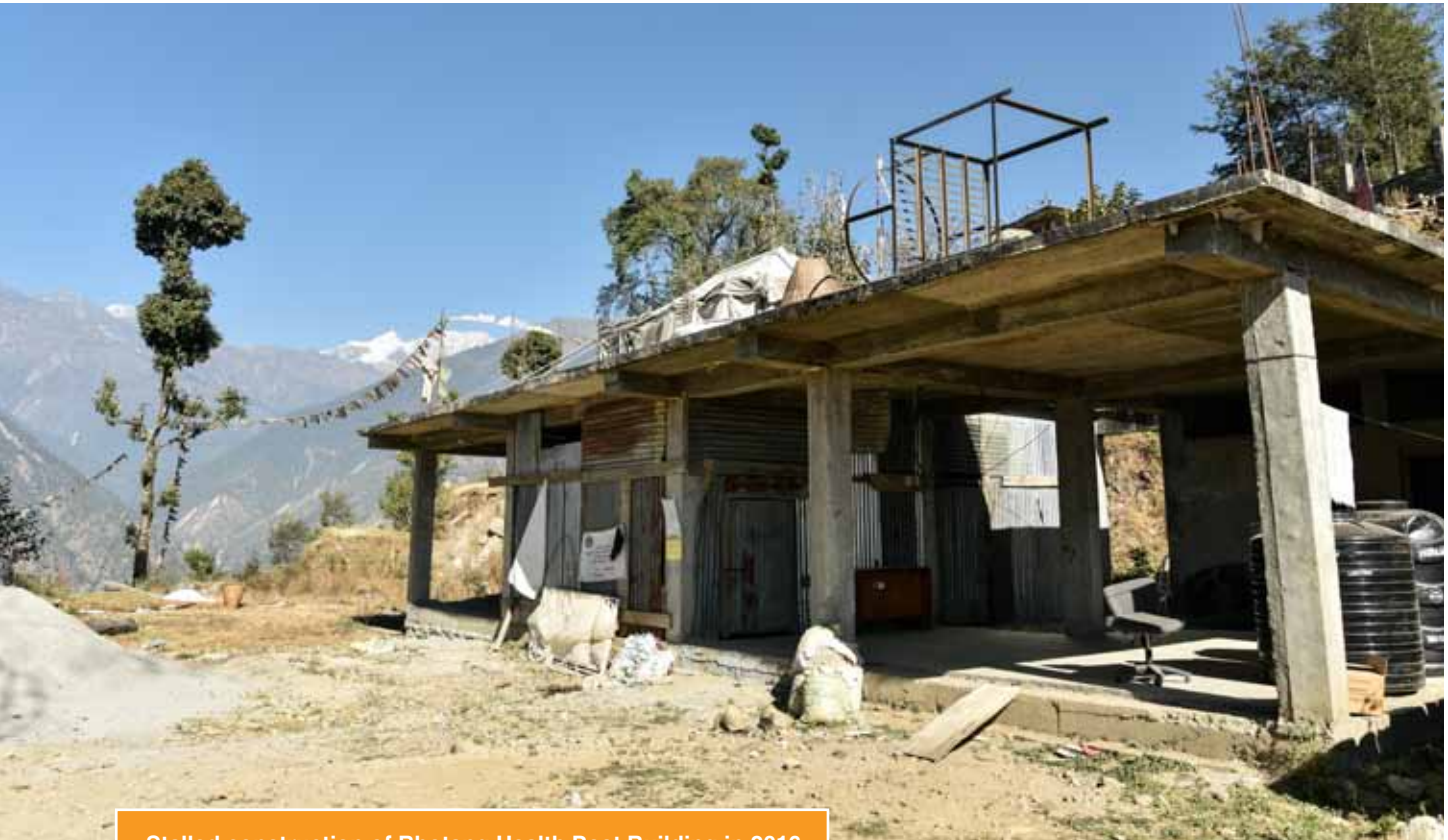
Stalled construction of Bhotang Health Post Building in 2016
