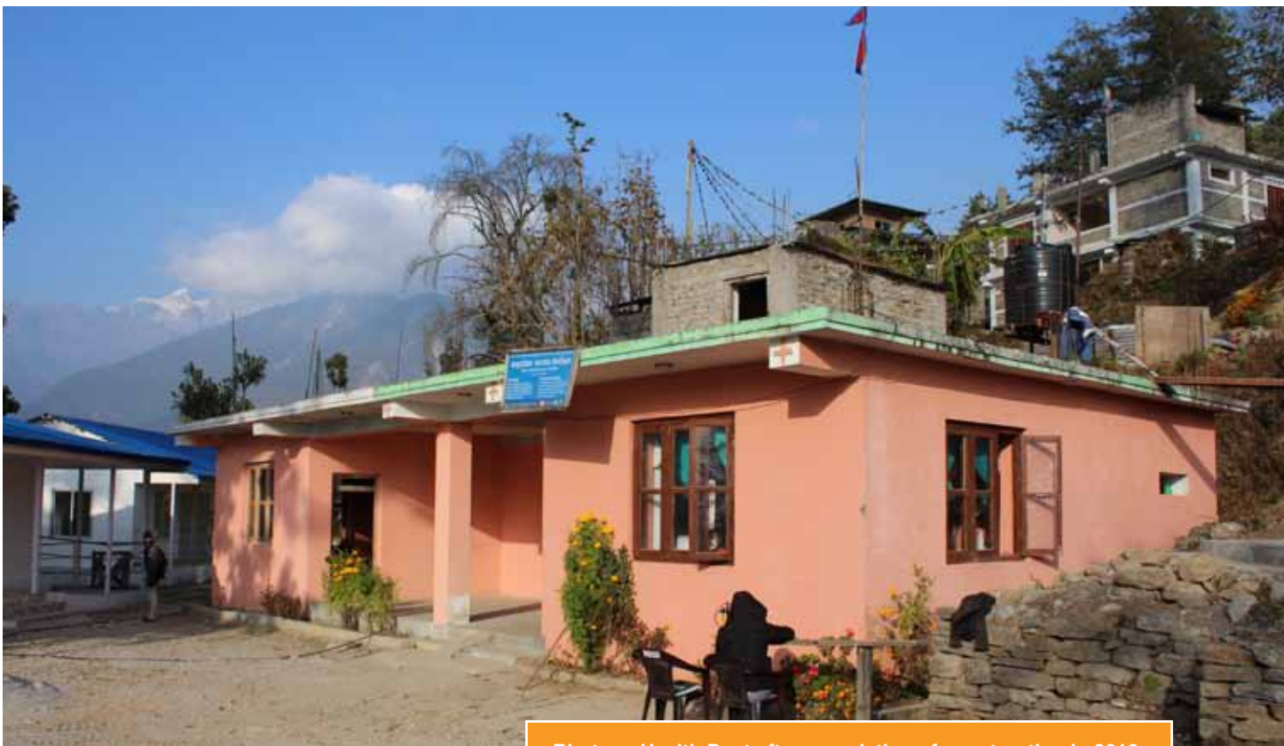
Bhotang Health Post after completion of construction in 2018
