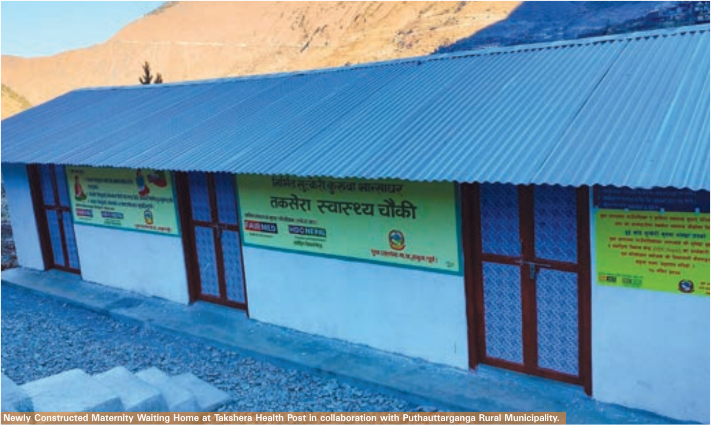
Newly Constructed Maternity Waiting Home at Takshera Health Post in collaboration with Puthauttarganga Rural Municipality.
